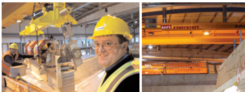
Above: Dr Nick Terrill, Principal Beamline Scientist, overseeing the installation of the first girder, carrying vacuum equipment and magnets, into the storage ring
