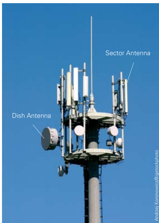
Figure 1 Two types of antennae at a mobile phone base station. Each type both transmits and receives RF radiation.
