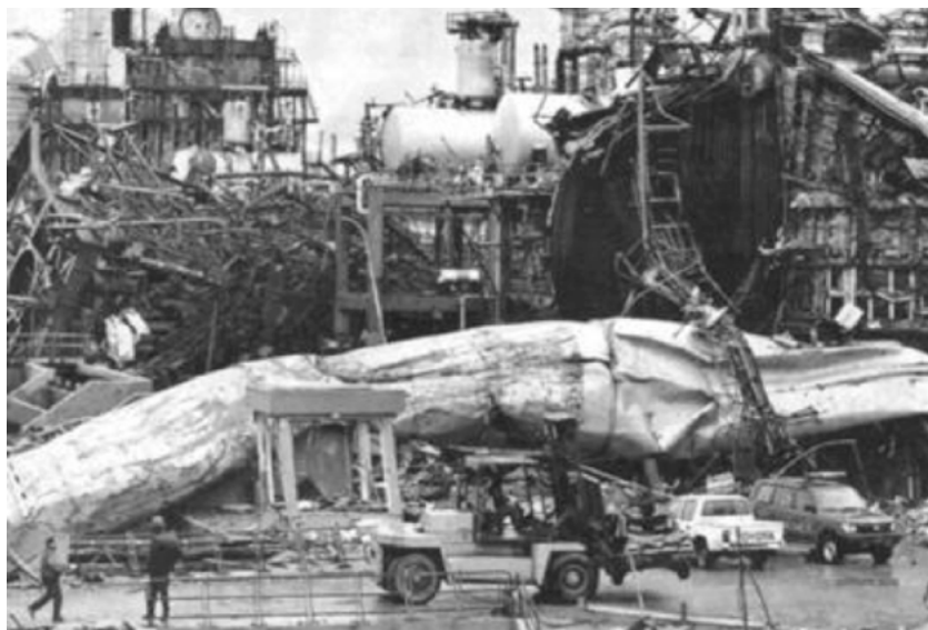
The Skikda liquefied natural gas plant in Algeria was destroyed by an explosion caused by mercury corrosion.
