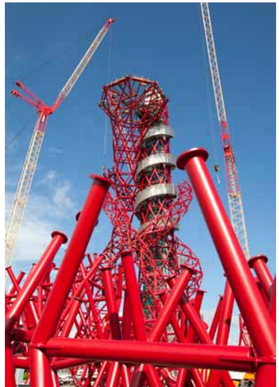
2000 tonnes of steel and 19 000 litres of paint have been used to build the ArcelorMittal Orbit tower
