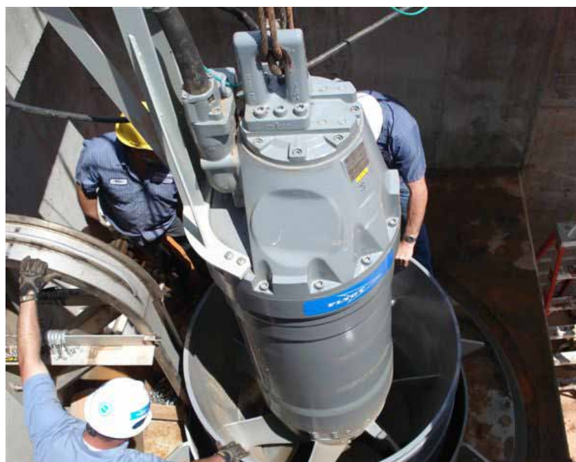
A pump being lowered into position
