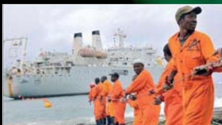
Bringing a SEACOM link cable ashore from the cable-laying ship.
