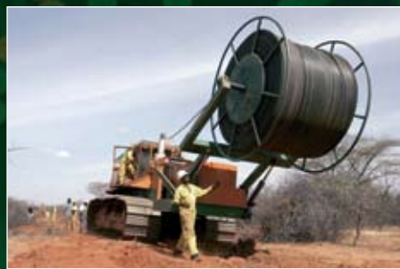
Laying the cable across rural Uganda.
