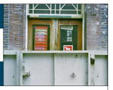
It works like a moveable barrier, it physically stops the water from entering the property.
