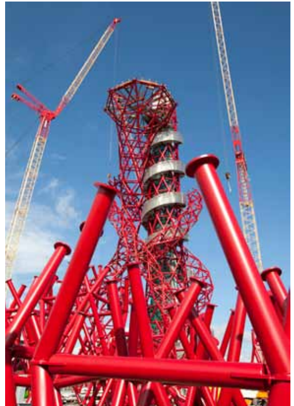
2000 tonnes of steel and 19 000 litres of paint have been used to build the ArcelorMittal Orbit tower
