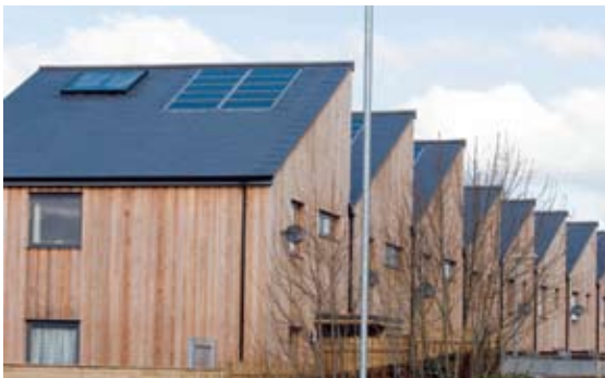
Houses with both solar water heating and PV electric panels at Primrose Hill Solar Village, Huddersfield. This development of 121 homes was part of a regeneration scheme, reducing fuel costs for tenants as well as greenhouse gas emissions. Some of the houses were refurbished, resulting in significant savings of emissions when compared to new buildings.
