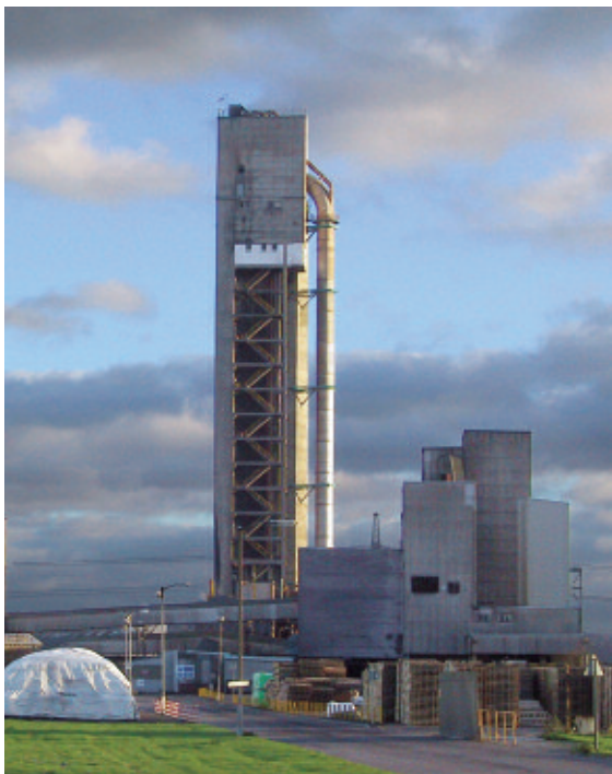
Right: A prilling tower
