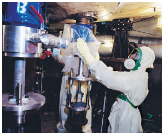
Workers underneath the main part of the Windscale advanced gas cooled reactor removing parts that might be contaminated
