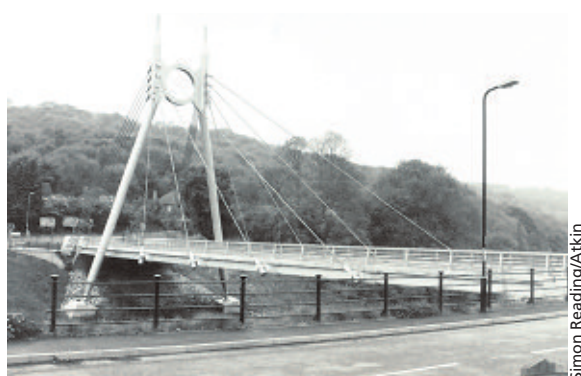
A bridge at Ironbridge designed by Simon. The river banks are shifting and the foundations had to be built so that one side took all the load.
